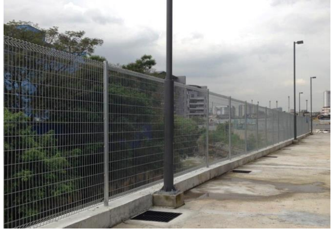
Anti Climb Perimeter Fencing
